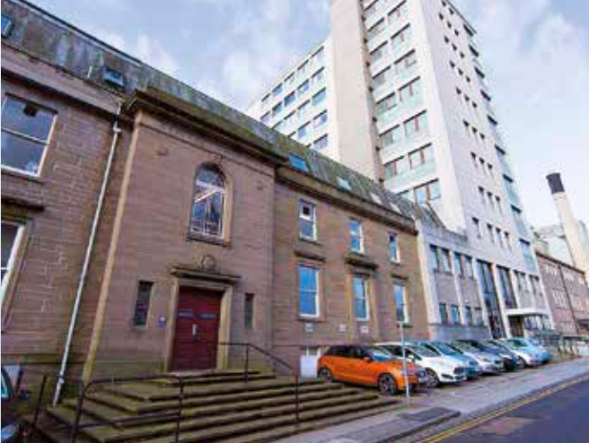
Fig 5 – Dental hospital and school complex photographed in 2015, showing the old hospital building (1954) and new tower (1968)
