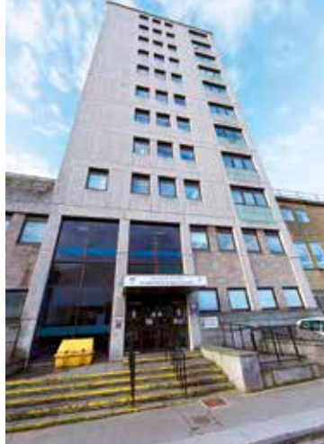
Fig 6 – The entrance to the modern dental tower. Clinics are located on the first five floors, lecture/study facilities and board room on the sixth floor. Floors seven to 10 inclusive are for teaching, staff offices and research labs
